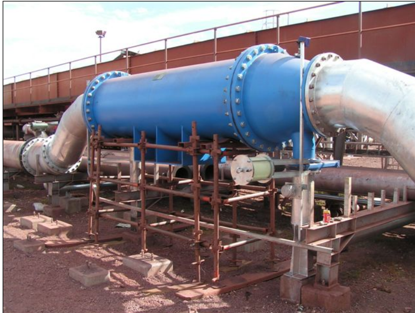
Figure 2: Screen Installation - Sishen Mine
